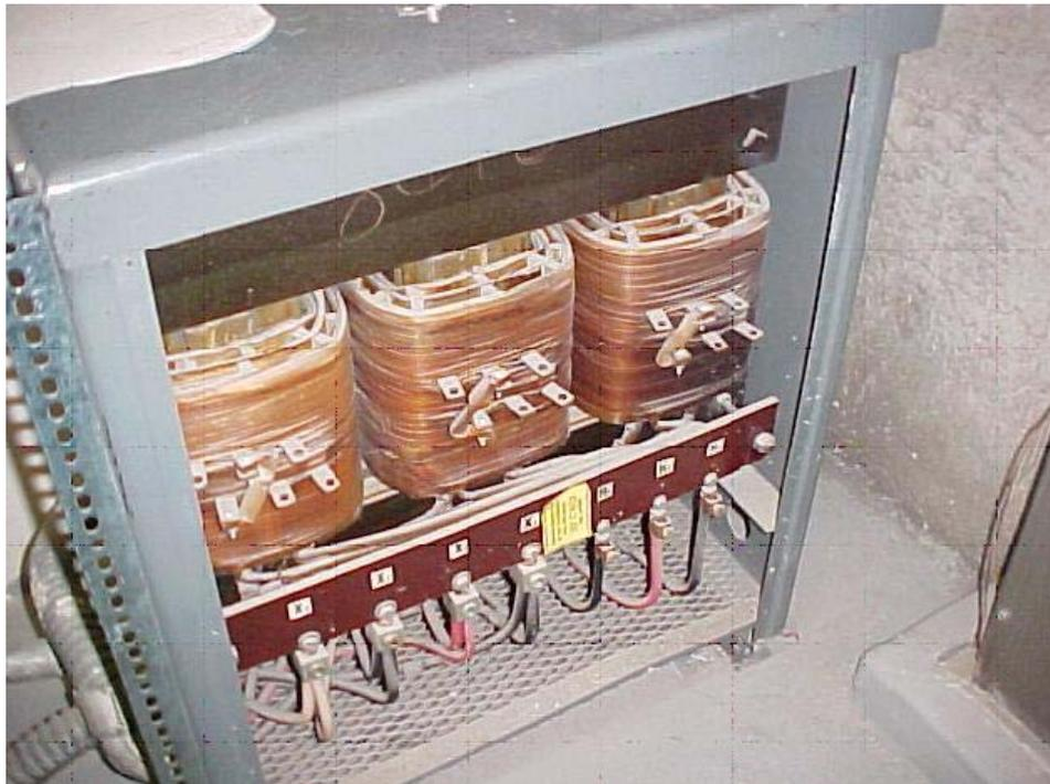
**Photo 2 – Photograph of 5<sup>th</sup> floor 75kVA transformer shown in photo 1 thermogram.**
